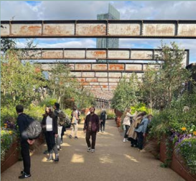
Castlefield Viaduct, Manchester
