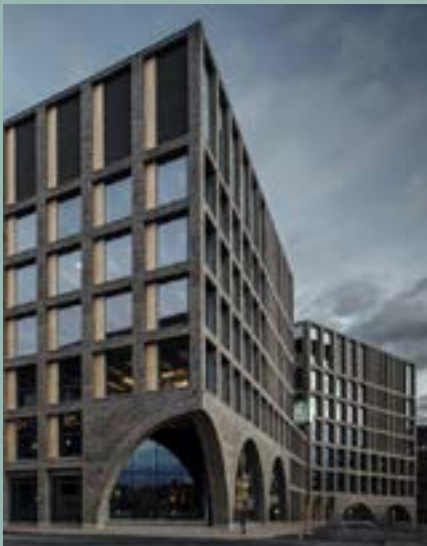
Urban Environment House, Helsinki
